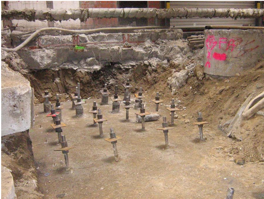
Figure 12. Finished micropiles
