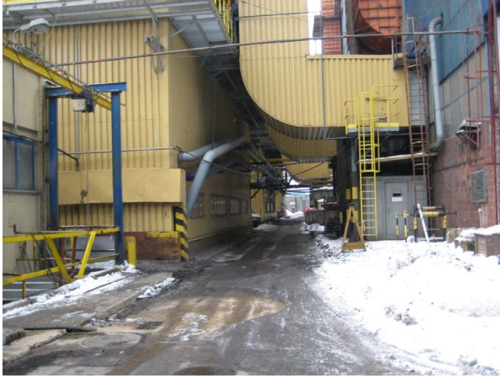
Figure 3. The same area seen from the ground level
